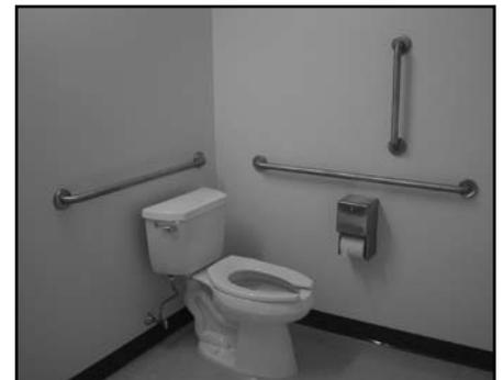
**Prisoner's toilet room:** The toilet room met all but one accessibility standard. The toilet paper dispenser was too close to the front edge of the commode and needed to be repositioned as required
