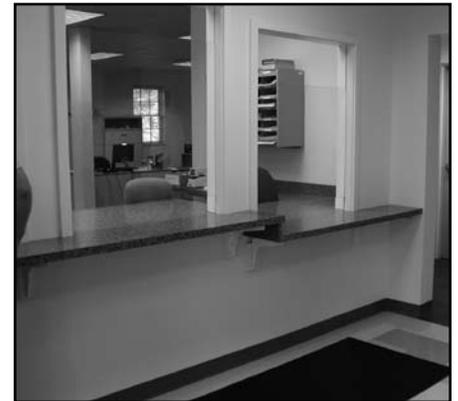
**Clerk transaction counters:** The accessible counter is seamless integrated into the overall series of clerks' counters
