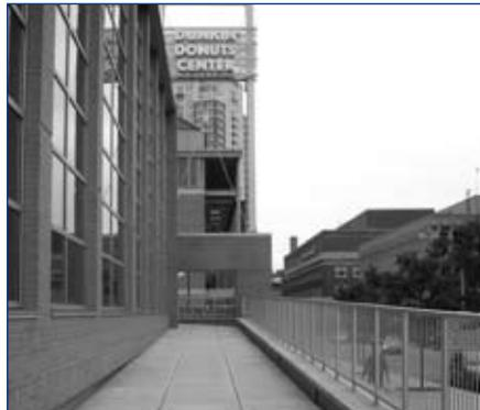
In addition to the pedestrian bridges, accessible ramps were created on the outside of the building as well as on the inside. With regard to the latter, the ramps up from the concourse to the arena were regraded to conform to the ADA.
