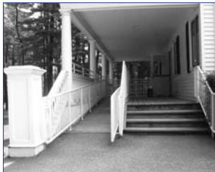
New ramp & stair at former enclosed side porch creates a new accessible entrance to the first floor level at Baxter House
