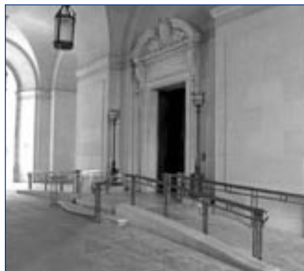
The ramps at this historic federal building were designed to provide equal access while preserving the building's original fabric.
